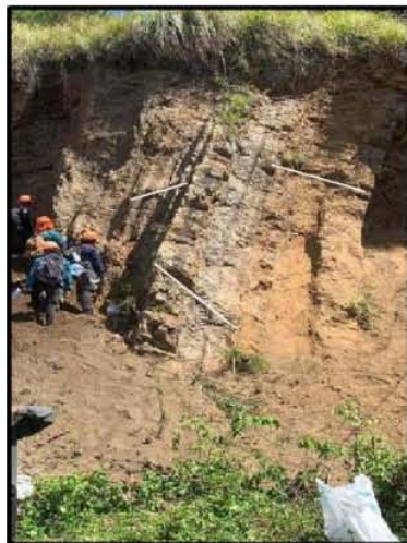
Figure 1: Outcrop with the position of the layers in the direction of the slope.
